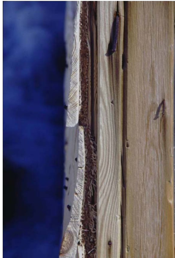
Figure 2: Details of Insulation, Cape Evans Hut. Adam Wild 2001
